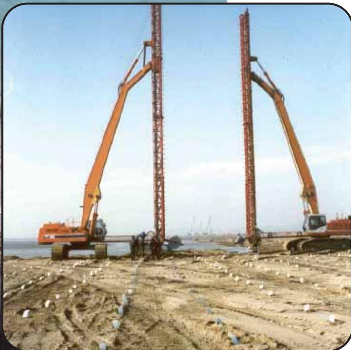
Thanks to its high performance Colbondrain is often the chosen PVD for major, technically demanding projects, such as the third runway at Changi Airport, Singapore. In this project Colbondrain has been installed to depths of up to 50 meters. The project required a total of 60 million linear meters of PVD and is probably the largest vertical drain reclamation project in the world.
